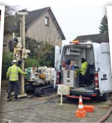
Week 3 Grondboringen Gerwen
